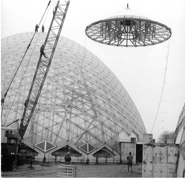
Figure 3 Photograph of the apex installation at the top of a dome. (Milwaukee County Parks Historic Photograph Collection)
