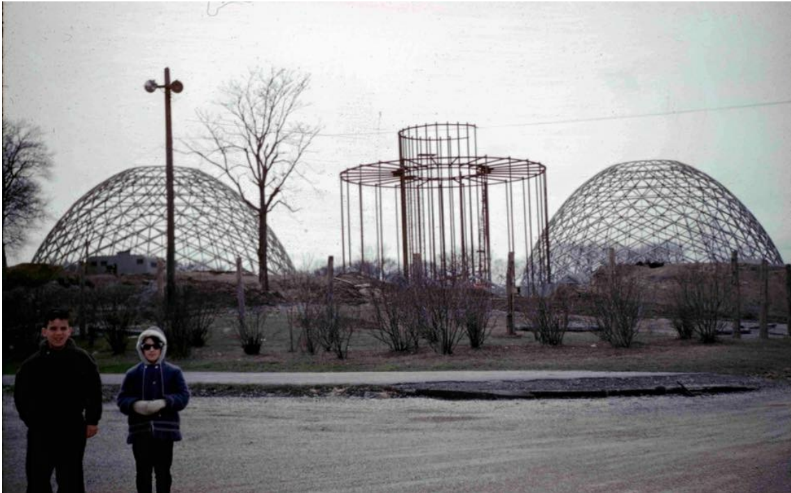
Figure 7 Photograph of the falsework used to construct the Arid House. (Milwaukee County Parks Historic Photograph Collection)
